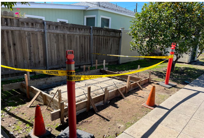
Construction has begun on the display shed and the shade trellis.
